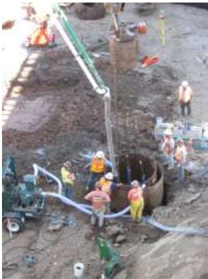
Pouring footings for the shoo fly. The right picture marks the point where the old/temporary bridge will touch land.
