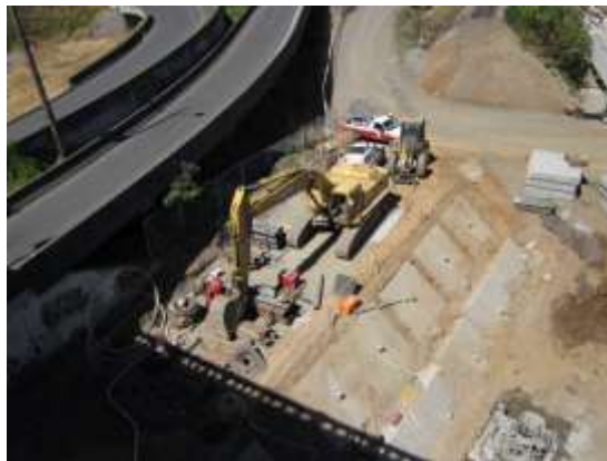
Pouring footings for the shoo fly. The right picture marks the point where the old/temporary bridge will touch land.
