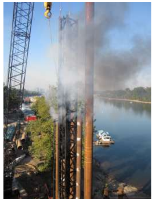
New pilings being driven
