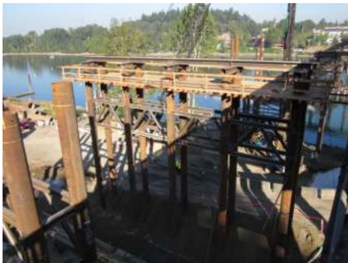
Supports for the temporary bridge are taking shape
