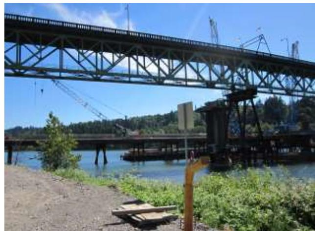
The low bridge is the temporary construction bridge. When complete, it will have to hold the weight of the biggest cranes
