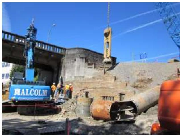
Work on the east side is to strengthen the bridge abutment before the eventual installation of the main bridge footings.
