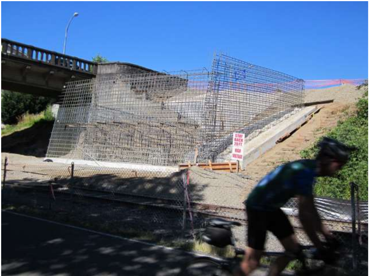
Rebar reinforcement cage for the concrete footing of the east side landing of the bridge
