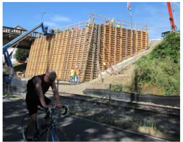
Concrete pour for the eastside bridge landing
