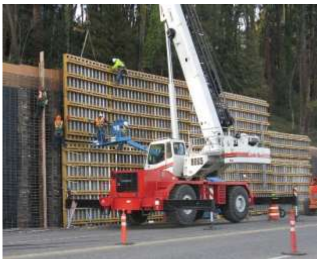
Placing forms for wall fascia
