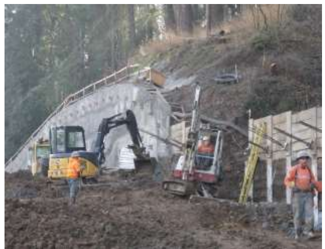
Excavating west retaining walls
