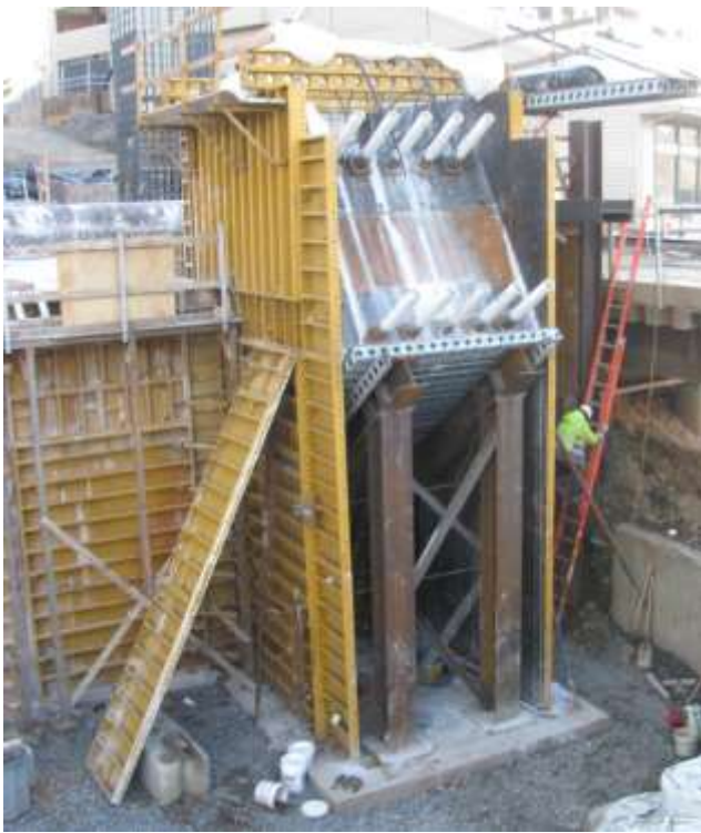
"Angel Wing" at Bent 6 after pour
