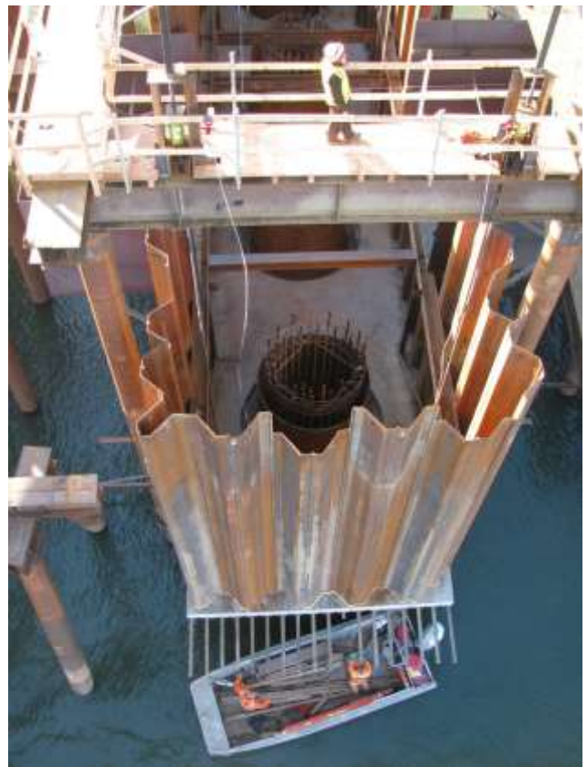
Lowering perched box caisson
