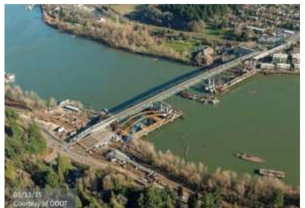
Sellwood Bridge construction Feb 11, 2015. Note the first set of steel arches in place on the west side of the river. (Photo by Multnomah County)
