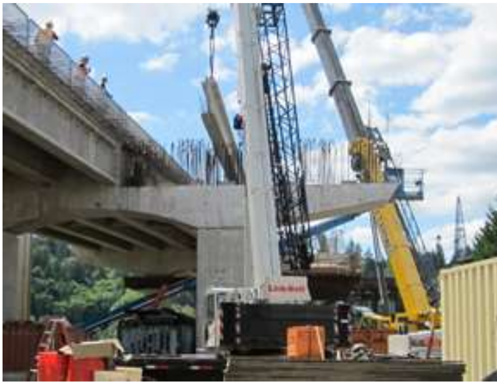
Concrete girder being lowered into place.
