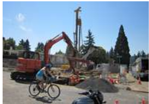
Massive drilling rig for the building foundations
